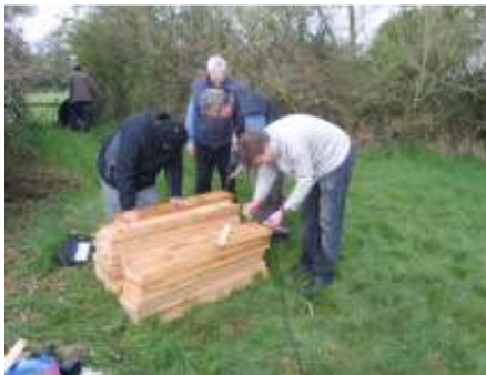
Cutting and drilling the timbers
