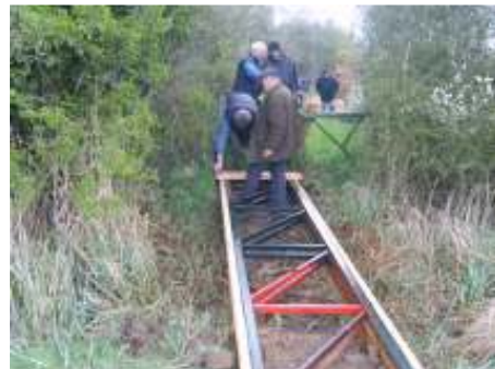
Laying the new timbers
